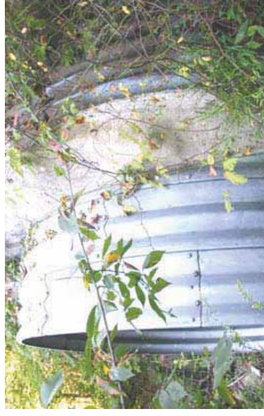
CMP liner in CMP host pipe with grouted annulus
