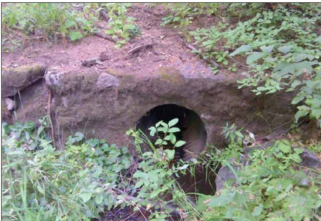
Figure 46. Photo. Light invert deterioration at inlet of CMP example on Mosquito Creek in Yosemite National Park.
