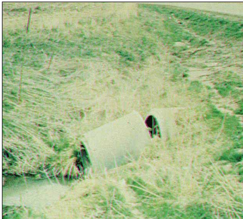
Figure 8. Photo. RCP culvert damaged by scour. (2)
