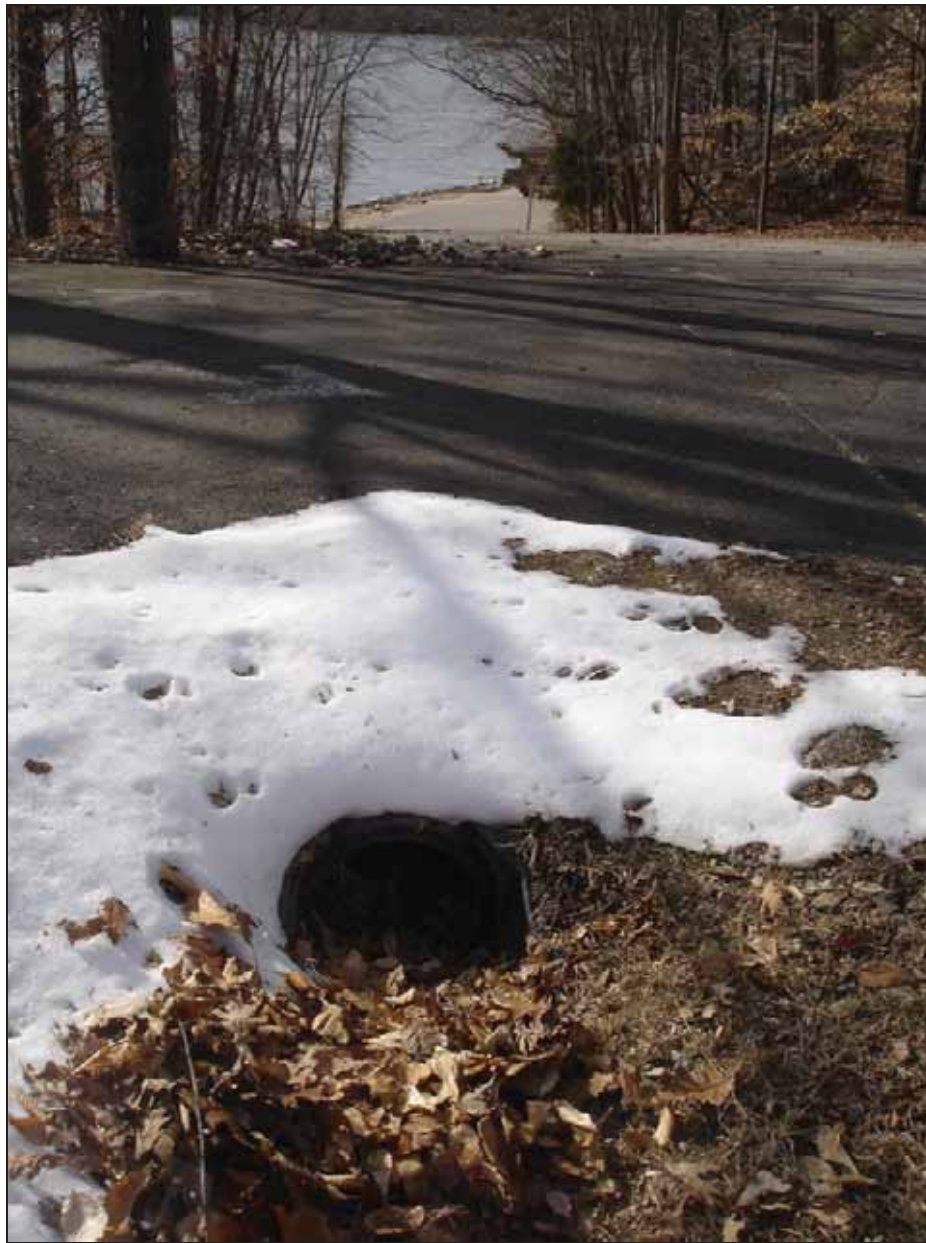
Figure 55. Photo. View of inlet of plastic HDPE example in Fountainhead Regional Park, Fairfax, Virginia.
