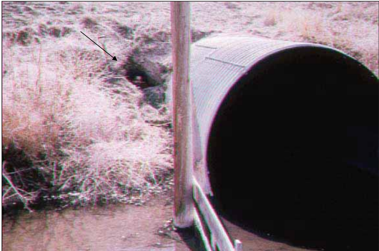
Figure 9. Photo. Example of piping through an embankment. (2)
