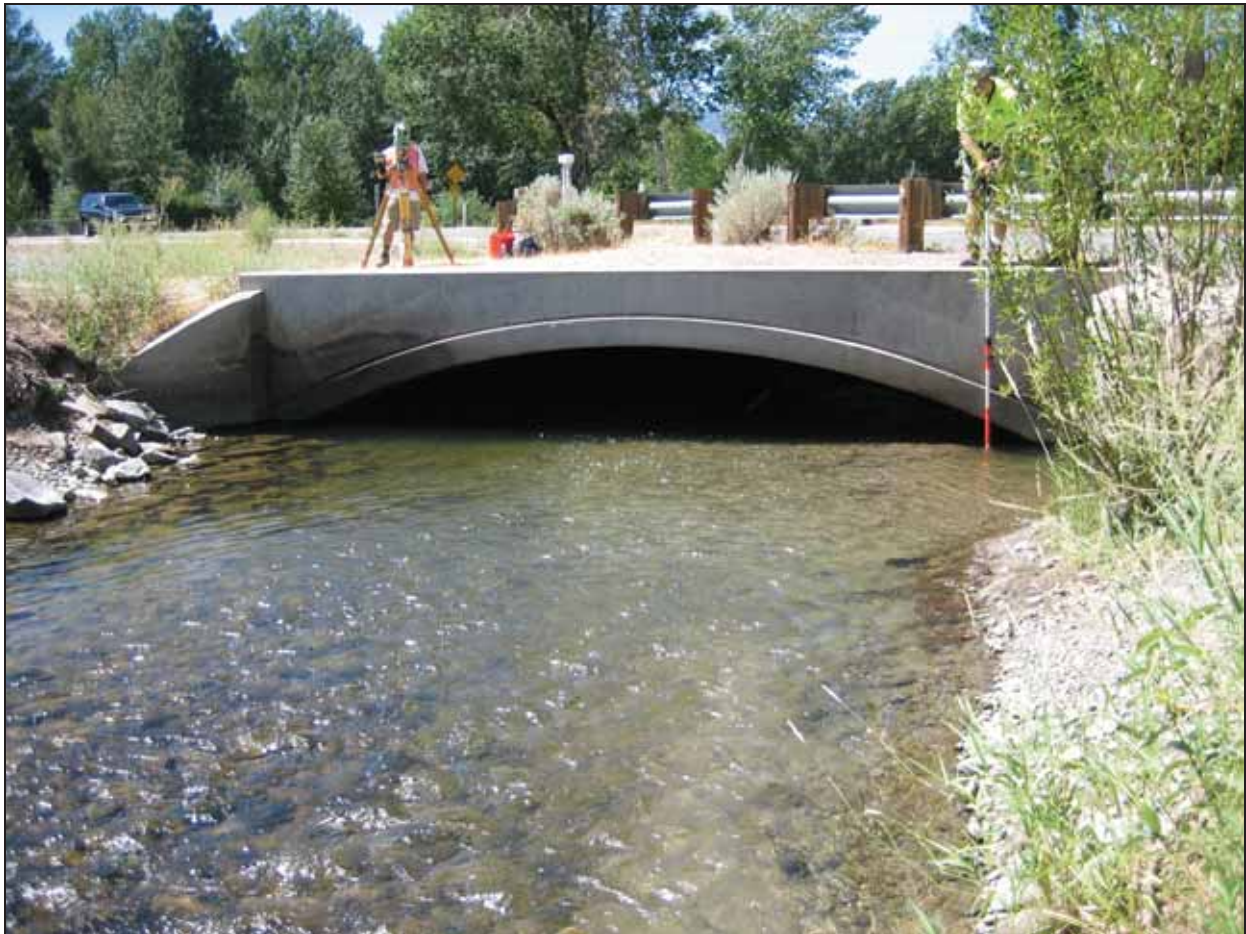
Figure 15. Photo. Example of an open-bottom culvert.
