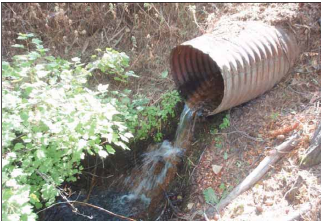
Figure 45. Photo. Light invert deterioration and minor local scour erosion at outlet of CMP example.
