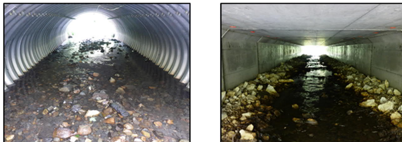
Figure 18: AOP structure without interior banks at Cabot Mack Mnt Rd (left); AOP Structure with interior banks at STP SCRP 8 (right)
