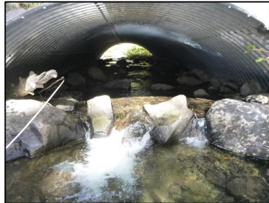
Figure 35: Rock sill at Middle Vinegar Creek
