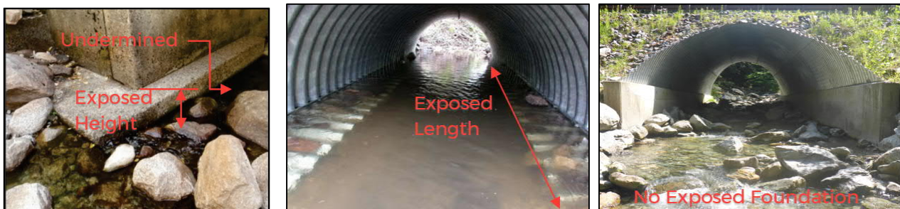
Figure 67: Exposed concrete spread footer measurement (left) 8 , exposed metal spread footer (center) 9 , and metal arch culvert on concrete footings with no exposed spread footer at White River
