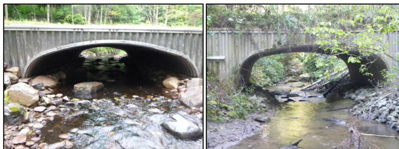
Figure 74: Large Roughness Features: Single, random boulders at Porcupine Creek (left) and bedrock, channel margin at Tottery Pole Creek (right)
