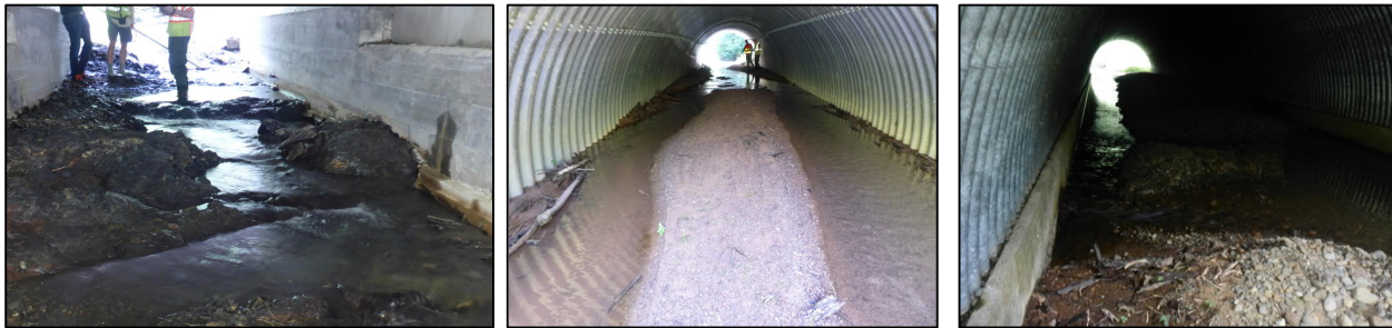
Figure 72: Flow Observations: Flow concentrated left wall at Marsh Brook (left), along both walls (split flow) at Saxine Creek (center), along both walls (alternating) at Tributary to Shafer Creek (right)
