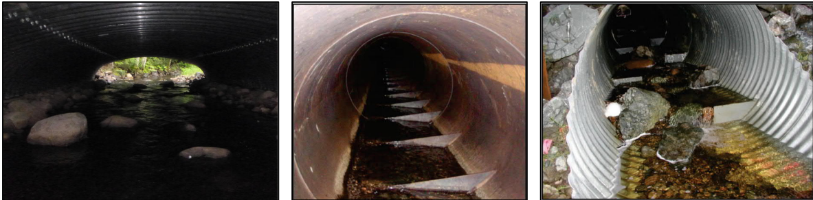
Figure 33: Random boulders at Porcupine Creek, WI (left); Baffles on channel margin 6 (center); Baffles in pattern 7 (right)
