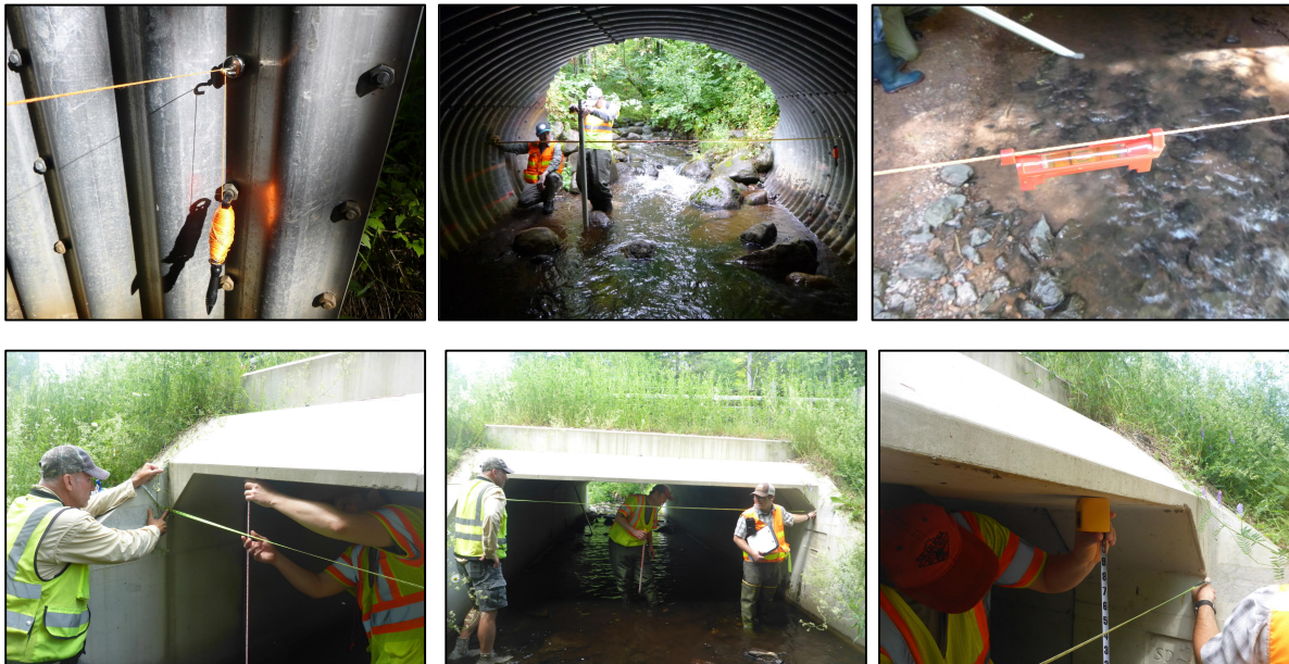
Figure 78: Using magnet hooks, two field staff measure the interior cross section at Pre-emption Creek (top); while three field staff take interior cross section at Howe Brook (bottom)
